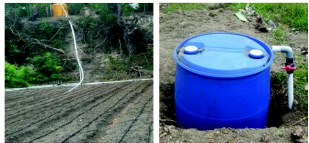
Instalasi sistem irigasi curah bergerak di lokasi food smart village (FSV) Noelbaki.
