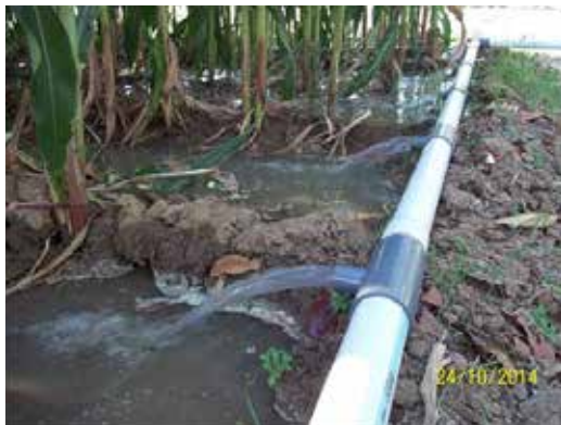
Gambar 2. Gated pipe furrow irrigation di KP Balit Sereal Maros
