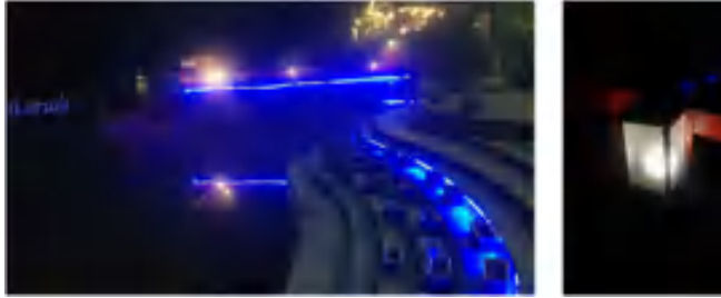
Figure 3. Perimeter illumination at the amphitheater and bridge at Teras Cikapunding in the form blue LED strip light, and bollard.
